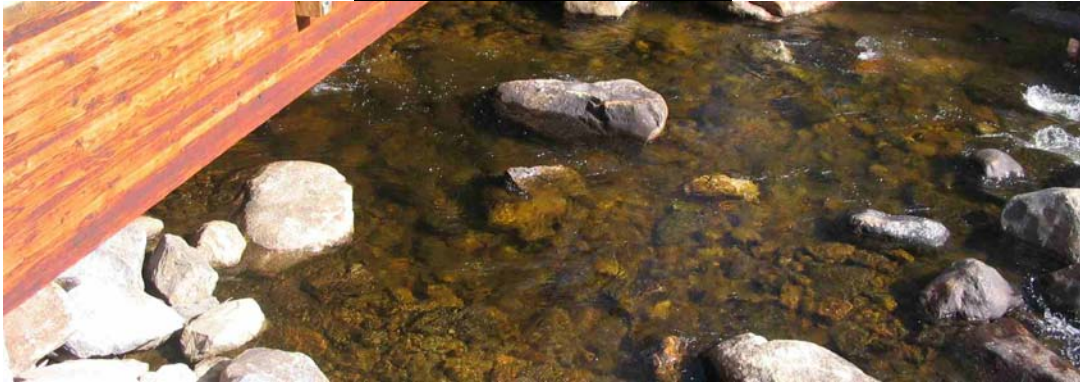
North Inlet under Grand Avenue Bridge (9/05)
